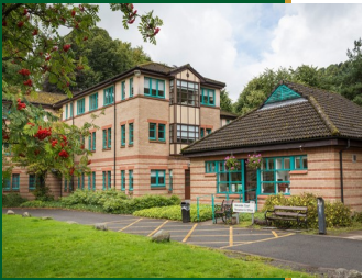
Alexander Court Flats
